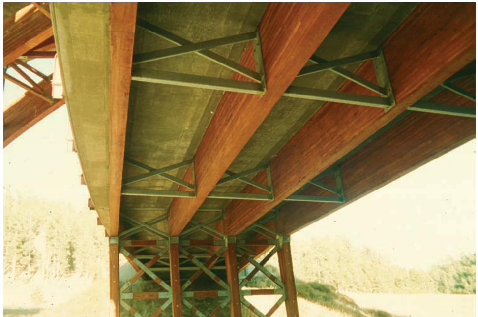
Figure 6.2.14 Glulam Beams with Numerous Fastener Locations
