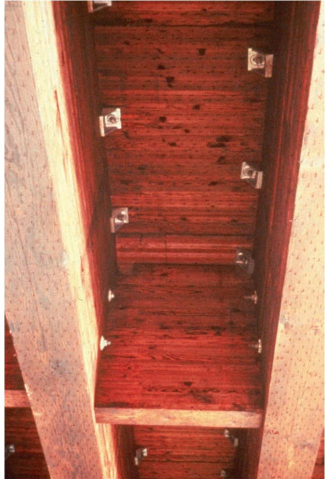
Figure 6.2.8 Typical Glulam Diaphragm
