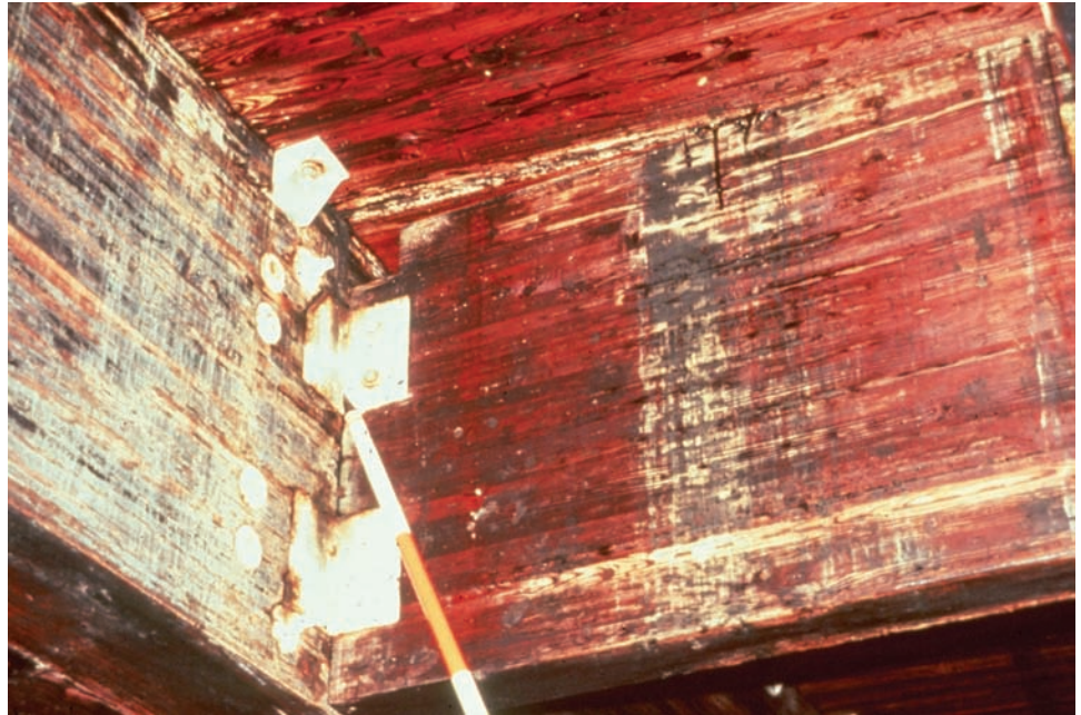
Figure 6.2.13 Typical Diaphragm for a Glulam Multi-beam Bridge
