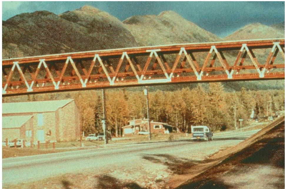
Figure 6.2.5 Parallel Chord Truss Pedestrian Bridge (Eagle River, Alaska)
