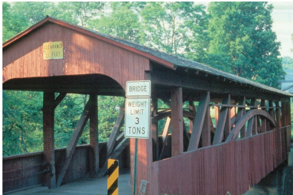
Figure 6.1.8 Burr Arch-truss Covered Bridge
