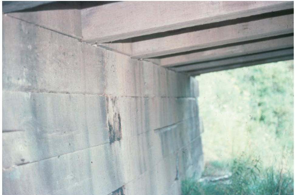
Figure 6.1.11 Bearing Area of Typical Solid Sawn Beam
