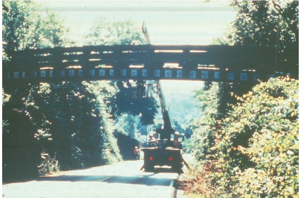
Figure 6.3.4 Glulam Stress-Laminated Timber Slab Bridge
