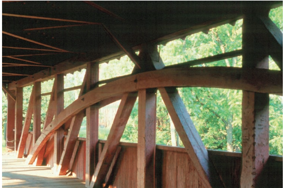
Figure 6.1.9 Inside View of Covered Bridge with Burr Arch-truss Design
