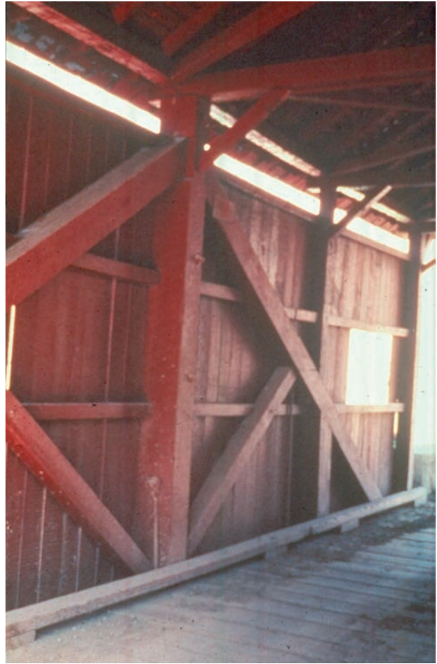
Figure 6.1.4 Inside View of Covered Bridge Showing King Post Truss Design
