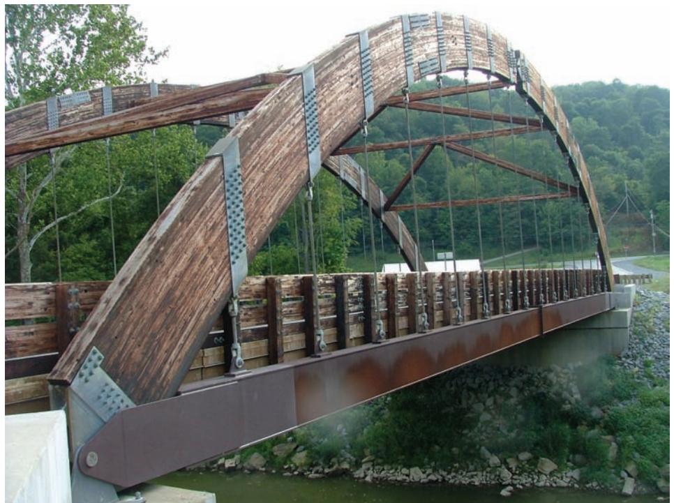
Figure 6.2.7 Glulam Arch Bridge (West Virginia)
