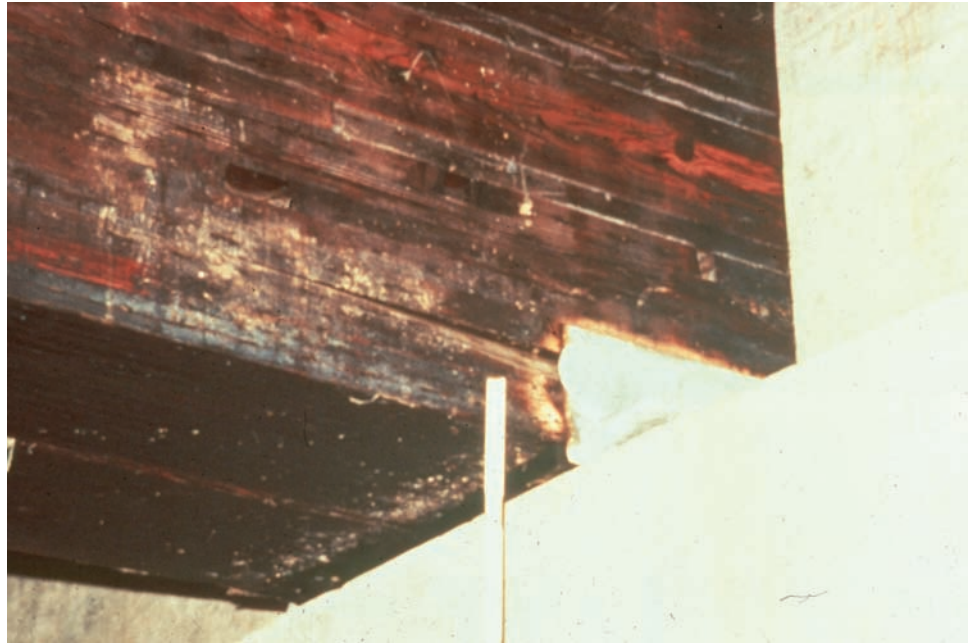
Figure 6.3.11 Close-up View of End of a Stress-Laminated Timber Bridge Showing Laminations
