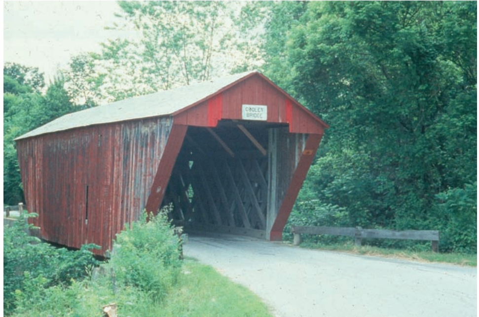
Figure 6.1.5 Town Truss Covered Bridge
