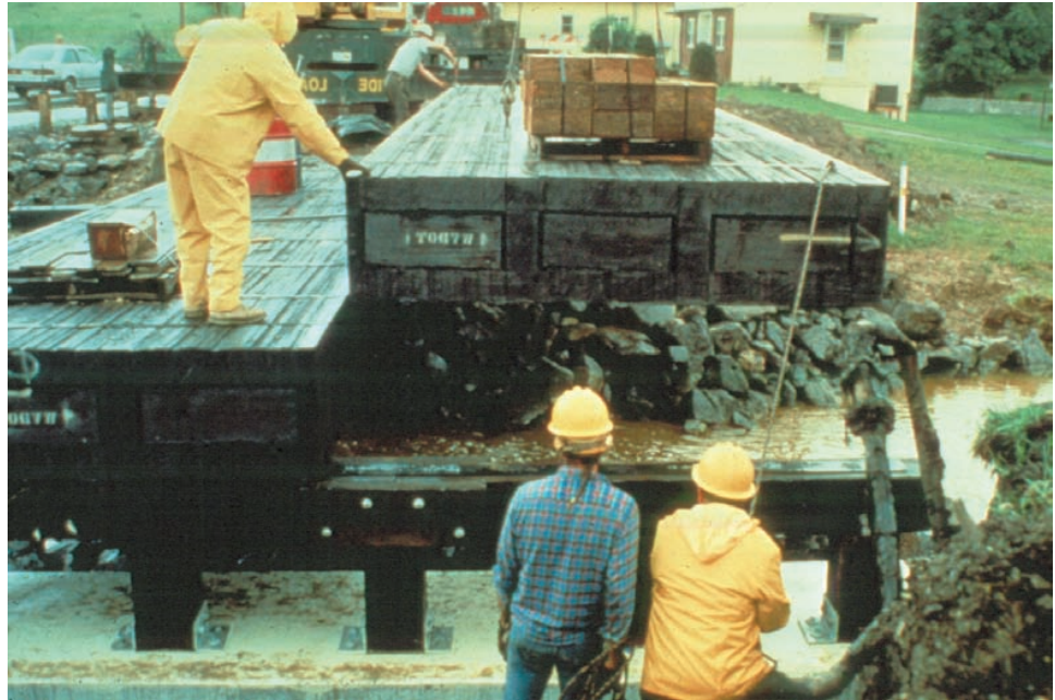
Figure 6.3.8 Stress-Laminated Timber Box Beam Bridge Being Erected
