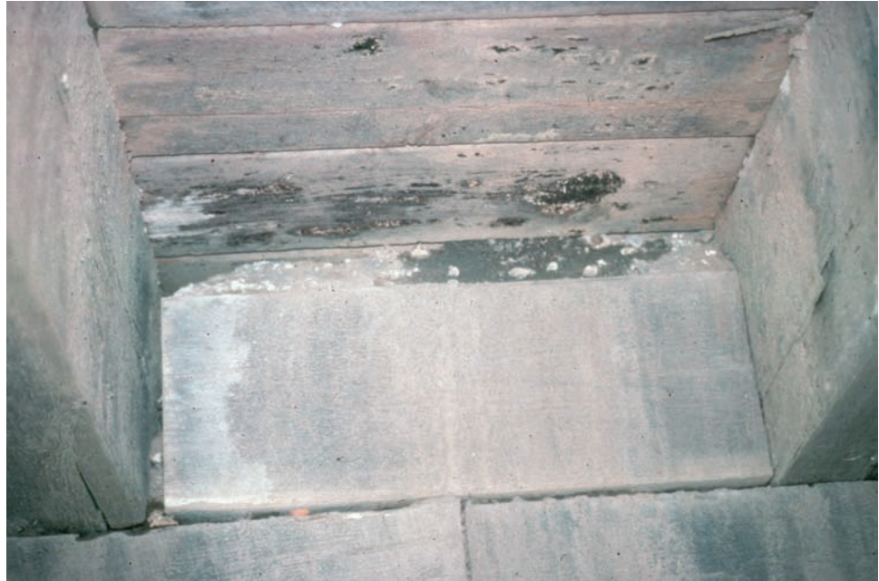
Figure 6.1.14 Typical Timber End Diaphragm
