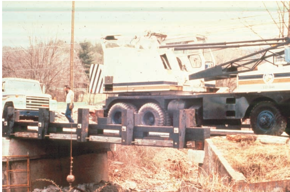
Figure 6.3.3 Stress-Laminated Timber Slab Bridge
